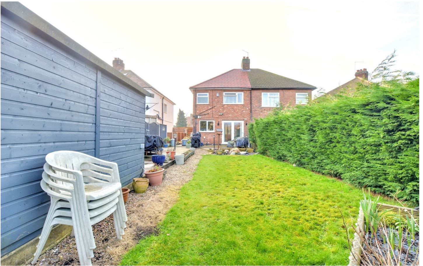
A traditional, bay-fronted, three-bedroom semi-detached house.
