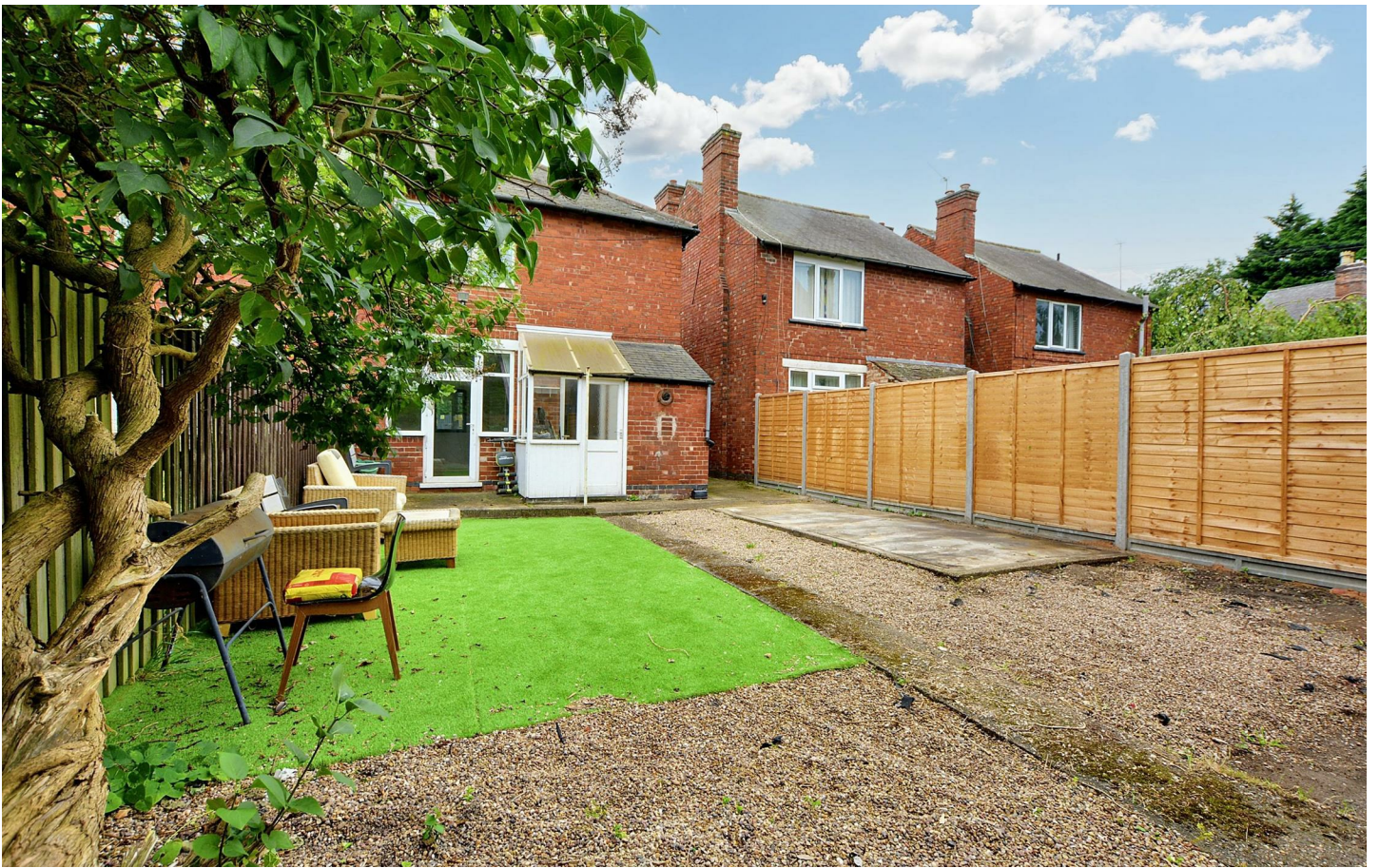
A traditional bay-fronted, three-bedroom, semi-detached house.
